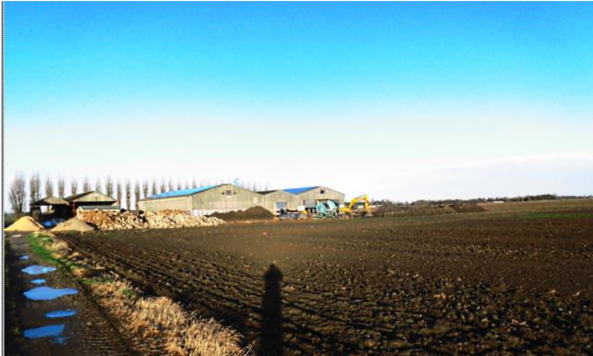
View from the east of Viner station looking west back towards the buildings
