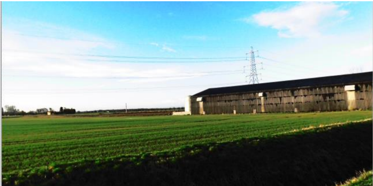
View from the east looking towards the south east elevation of the potato store
